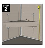
Hold the corner bench in place at an appropriate height (between 16" to 18" for suspended benches or 20" for diamond benches) from the shower base. For HYDRO-BLOK Suspended Benches, use a level to slightly slope the bench towards the front to allow water drainage.
