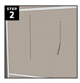
Locate and mark the locations of your wall studs so that the niche can be installed in the proper location. All HYDRO-BLOK niches must be installed so that they are supported by a stud on each vertical side.
